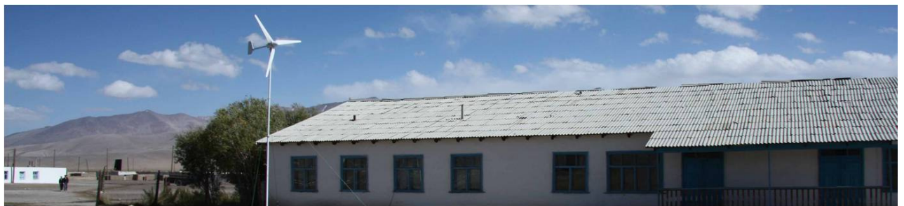
Turbine installation at Alichur school.
